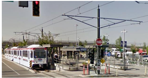
TRAX line, predictable MW-level pulsed load
